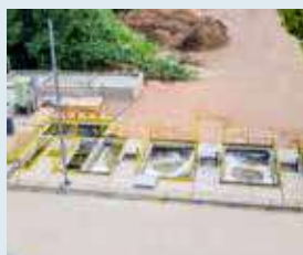
Water and Wastewater Purification
