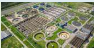
Industrial Water Treatment
