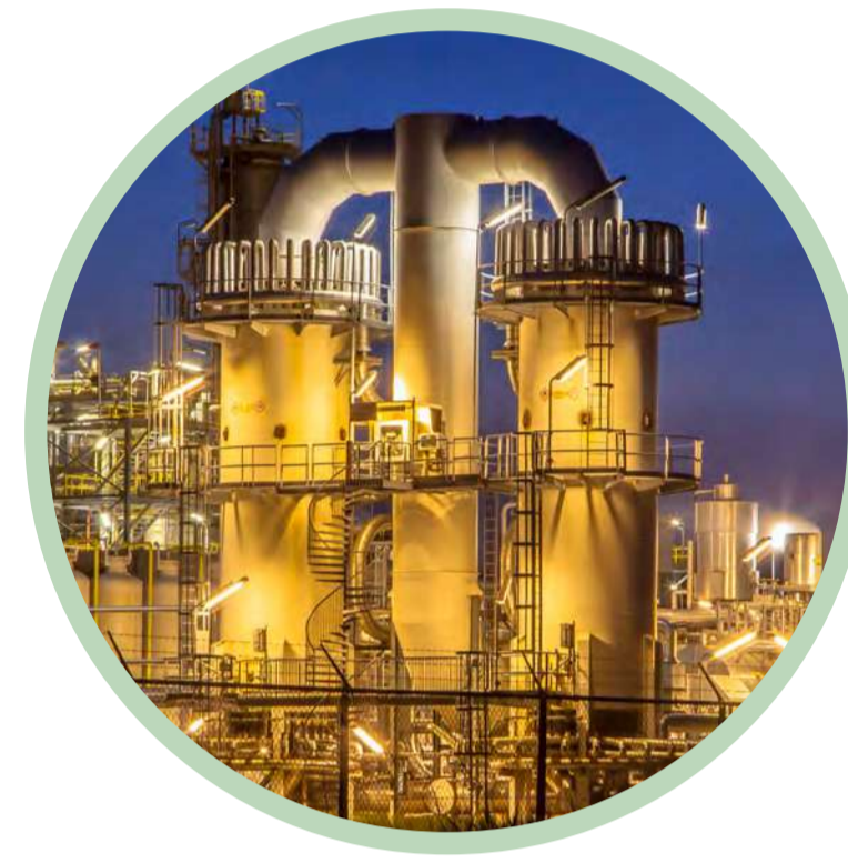
Chemical and petrochemical industries
